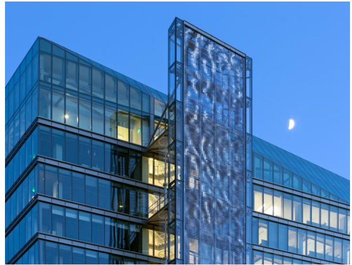
“Firefly” Ned Kahn, installed on the side of the Public Utilities Building at 525 Golden Gate Avenue. Funded by the 2% requirement. Photo provided by the San Francisco Arts Commission.
