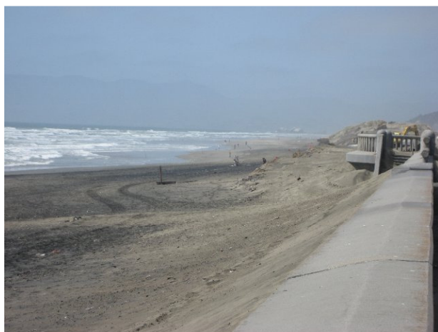
BEFORE: sand build-up on sea wall
