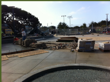
West Sunset construction in progress
