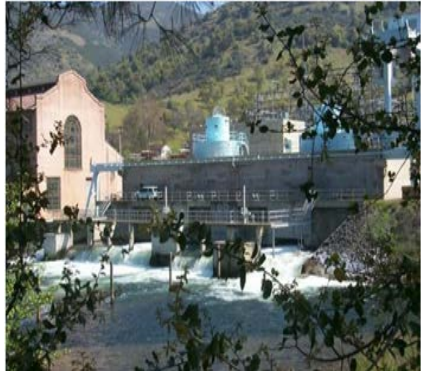
Moccasin Power House
