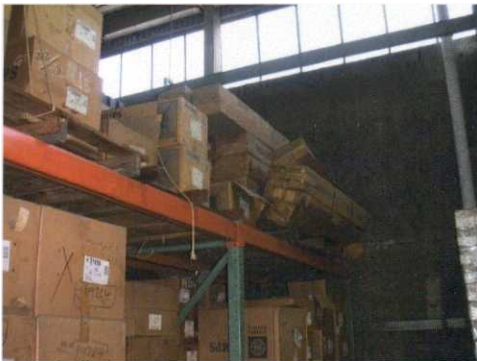
Photo 2 - Unsecured material storage on top rack, Main Storage Area/Supply room
