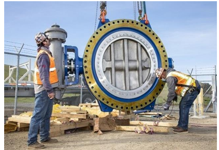
Removable Spool Piece (top); Butterfly Valve (bottom)
