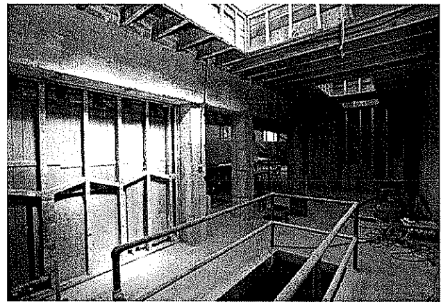
Golden Gate Valley Branch Library - Demo of New Workroom
