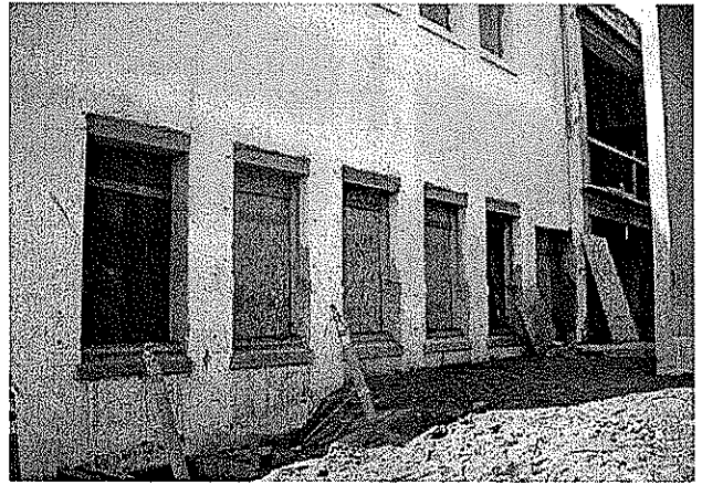
Anza Branch Library - Program Room Windows Slated to Open Winter 2011
