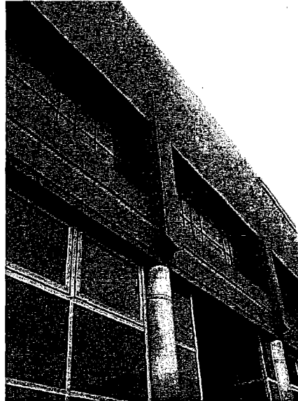
Second story, primary facade.
