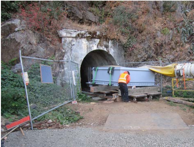
Moving the new bulkhead door frame into Adit 5/6
