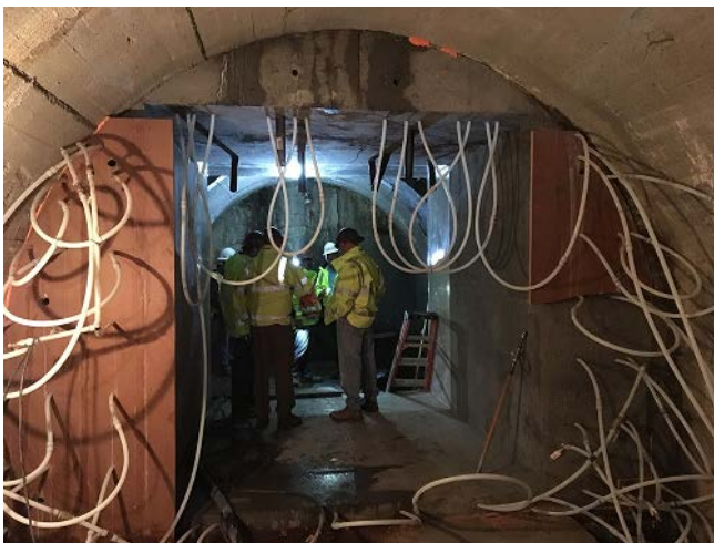
Removing the formwork from the new concrete plug at Adit 8/9
