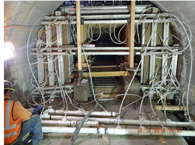
Chiller tube installation prior to concrete pour of new plug
