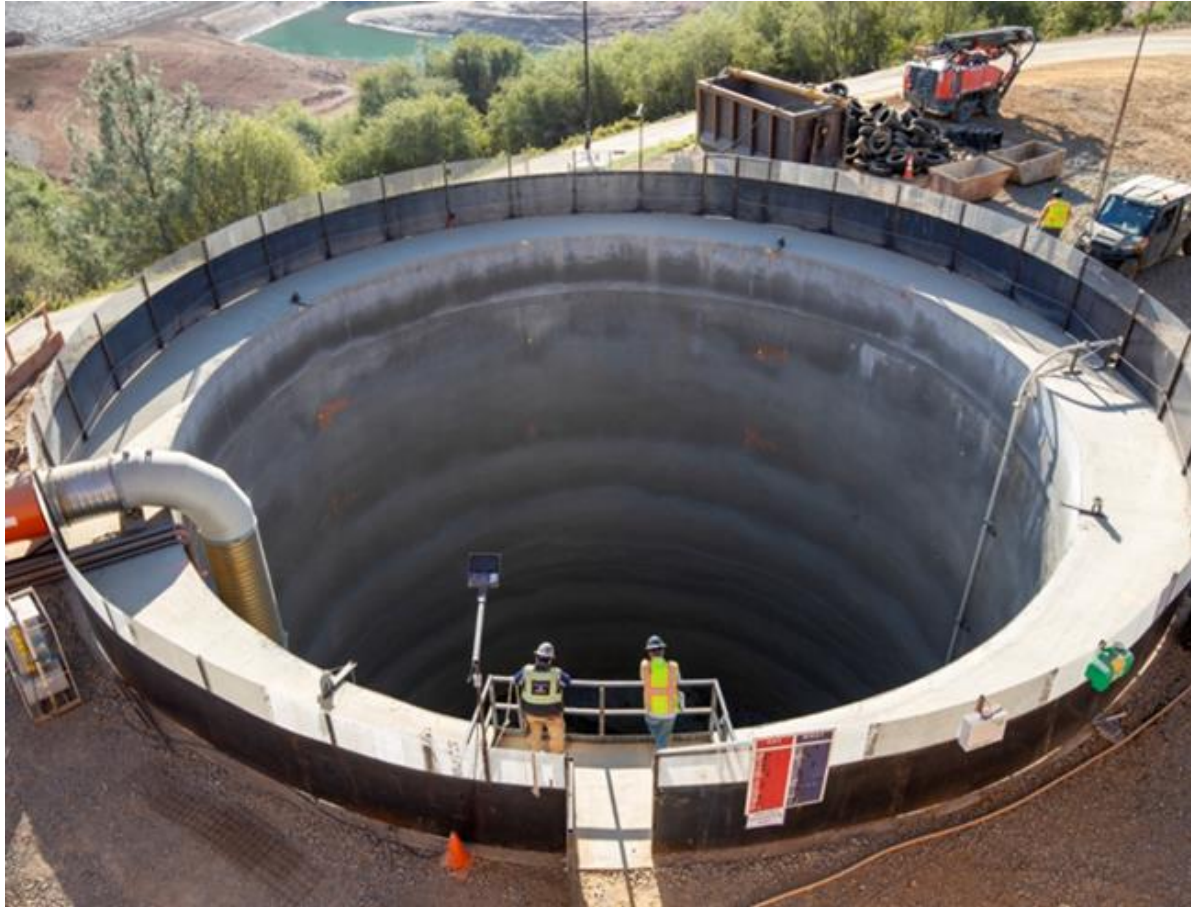
Flow Control Facility Shaft
