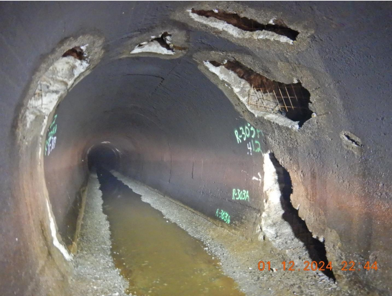
Tunnel Lining Repair
