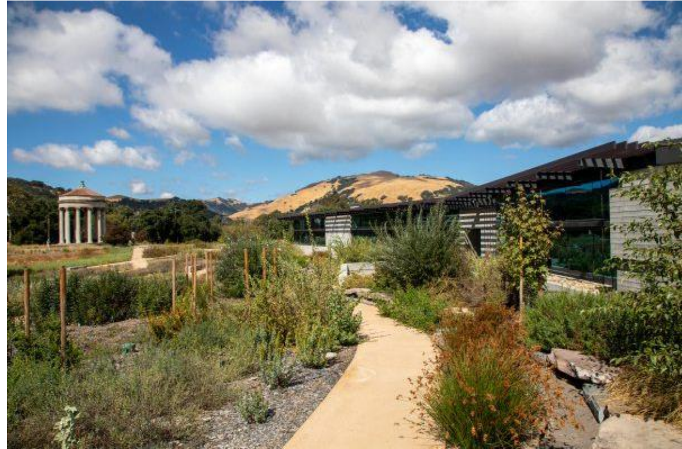
Phase 2: Alameda Creek Watershed Center
